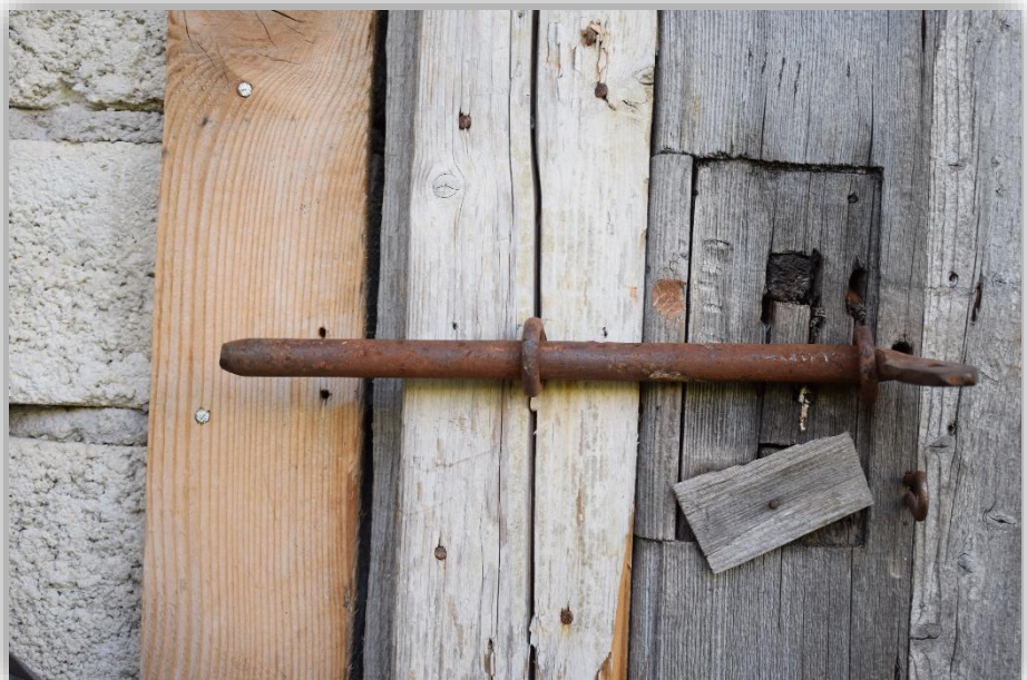
Figure 10. Chicken coop damaged on September 16 th and 17 th . It was a bear-proof structure but the door was the weak point: F1.99 just opened it just moving the latch (right picture). The owner avoided additional damages reinforcing the door.
