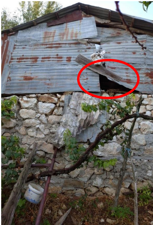
Photos 1 & 2: visible hole at the metallic “wall” of the pen opened by the trespassing bear (left) and livestock unit with poor construction materials (right).
