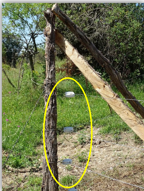
Figures 34-35. In the left figure, the e-fence is incorrectly installed, with the wire positioned on the inside of the corner wooden stake. In the right figure, one can see the grounding is improperly installed, reducing the fence's effectiveness.
