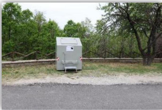
Figure 24. Installation of a bear proof metal shell at Pervali village
