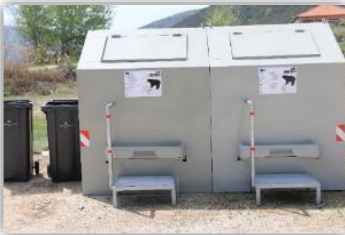
Figure 17. Installation of two bear proof metal shells at Pyli (National Park's Information Center)
