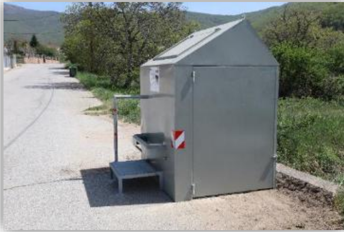
Figure 19. Installation of a bear proof metal shell at Lefkonas village
