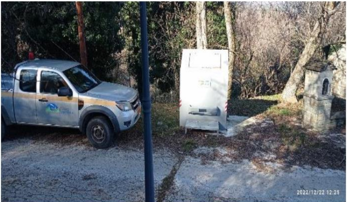
Figure 10. Installation of a bear proof metal shell at Kaloutas village
