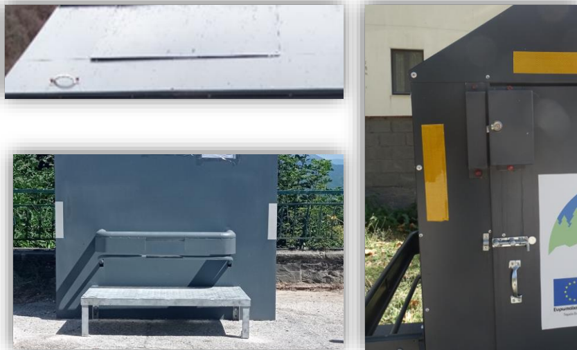
Figure 15. Modifications in the original scheme. Left above: the extra handle for better grip. Left bottom: the mechanism for the foot handle. Right the reflective strips and the lock
